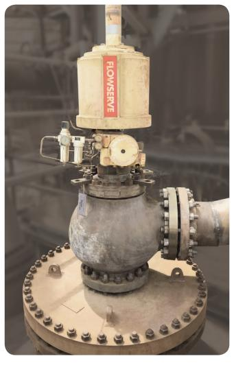
Valtek Survivor valve installed in flashing slurry letdown service
