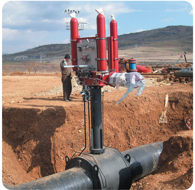
Welded body valve with extended stem
