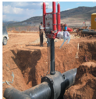
Welded body valve with extended stem
