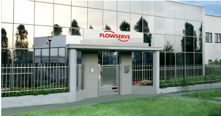
Flowserve Valbart Main Office
