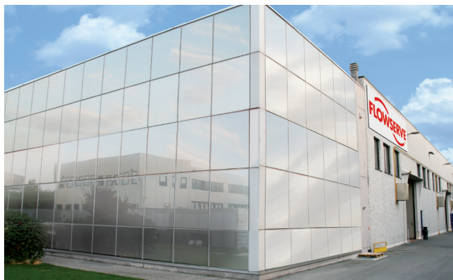
Flowserve Valbart Testing and VAC Centre
