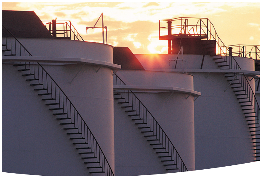
Auxiliary Card Being Installed
