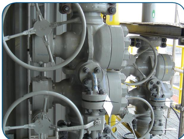
The valves illustrated are 6" class 2500 with hub ends, in carbon steel, manually operated.
